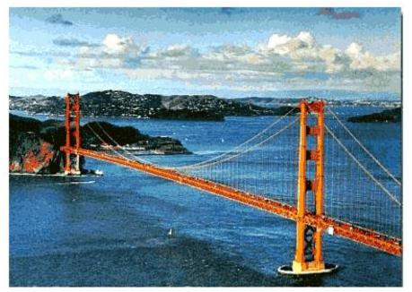
The cables of the bridge are parabolas. Let the vertex of one of the parabolas be (0, 0), the point at which the cable touches the side of the road. So the general form of the parabola is  $x^2 = 4py$ . We can solve for the equation of this parabola by substituting in the point (640, 160) – the height of one of the towers. Hence,
