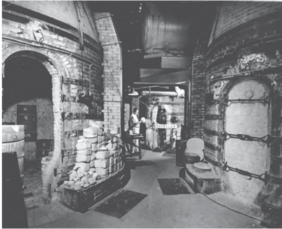
Interior image of the Rookwood Pottery factory
