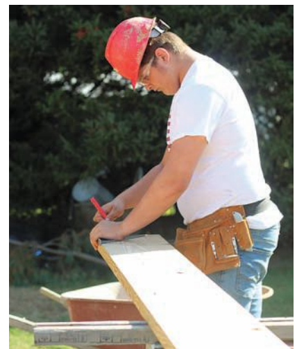
A student cuts a piece of lumber for the pole barn.
