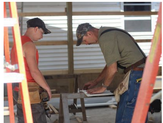
Gary Mitchel, right, shows a student how to cut siding for use on a pole barn the class built last spring.
