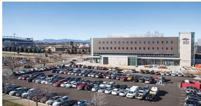
Metro State University’s new Advanced Manufacturing Sciences Institute, a $60 million collaboration between the university and Colorado employers.
